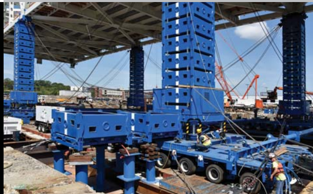
Beginning the lifting operations of new bridge from assembly site.
