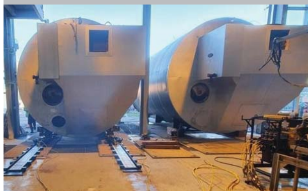
The boilers safely outside the boiler house.
