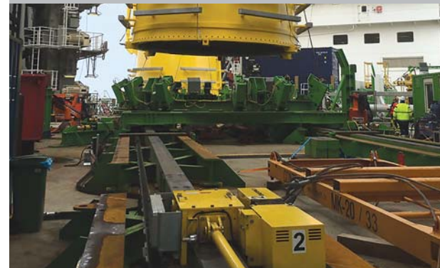
Loading of transition segments.
