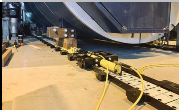
Preparing to skid the boiler out of the building.
