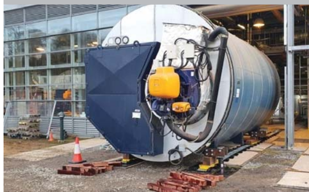
Boilers skidding in process.
