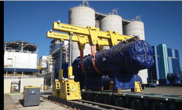
The Enerpac SL400 Gantry lifts the 138-ton high-pressure heater.
