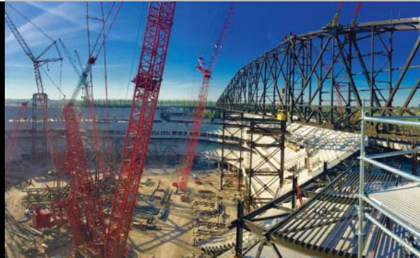
Enerpac SyncHoist system in use during roof truss picks.
