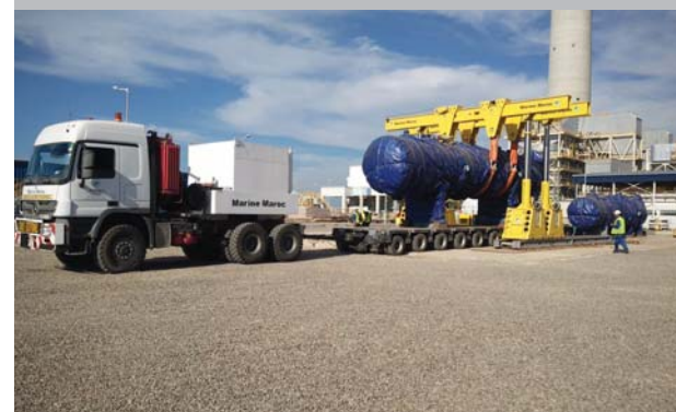
Lifting the high-pressure heater off the transport trailer.
