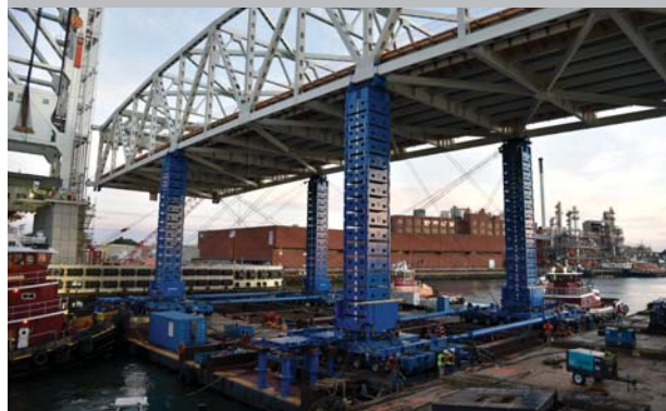
Positioning new bridge span into place.
