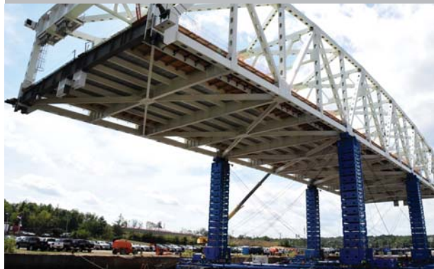
Fully lifted bridge ready for transport.
