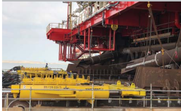
Enerpac ‘Push-Pull’ system for the platform module load-out.
