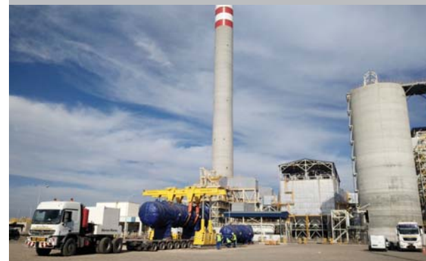
Delivering the high-pressure heater.
